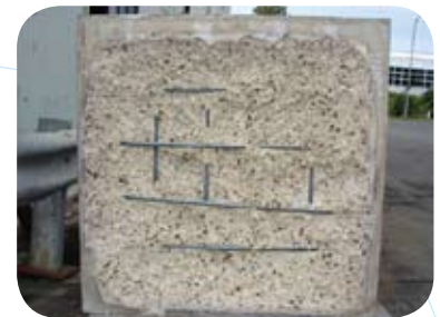
Damage to Specimen without BarChip F
